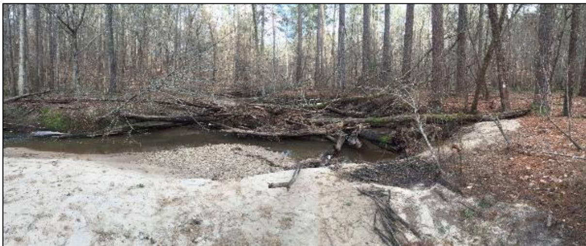
Figure 40. Debris dam of LWD, intermediate structure (Reedy Creek – Wake County, NC).
