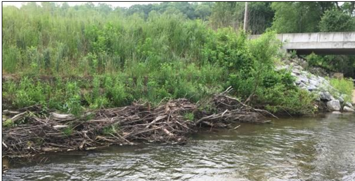
Figure 42. Toe wood structure a few years after construction.
