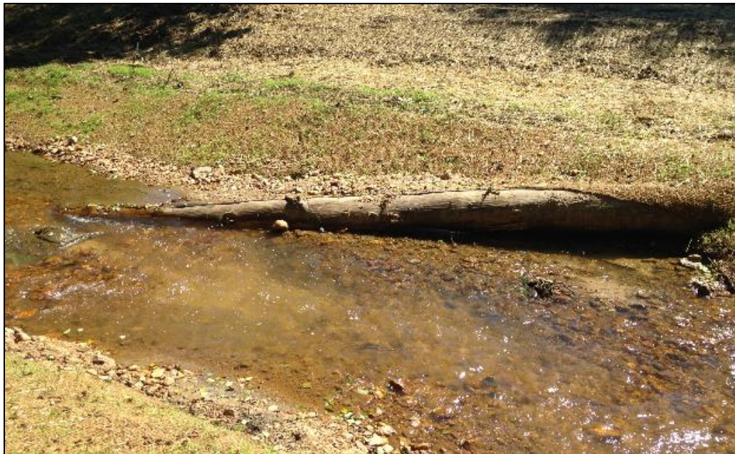
Figure 41. Log vane structure after construction.
